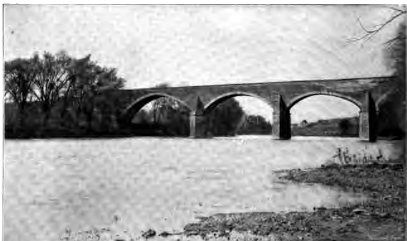
MONOCACY STONE BRIDGE. BALTIMORE PIKE
